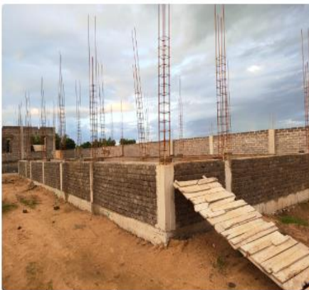
Under Construction Project
