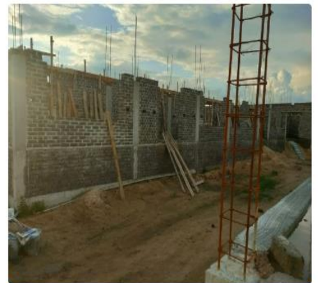
Under Construction Project
