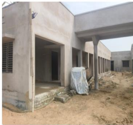
Under Construction Project
