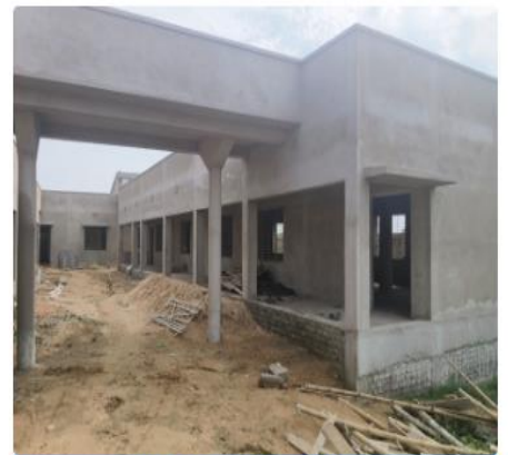
Under Construction Project
