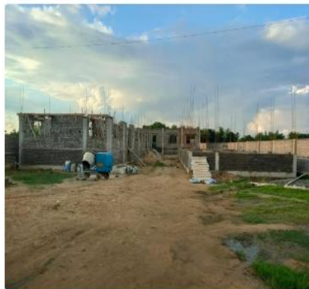
Under Construction Project
