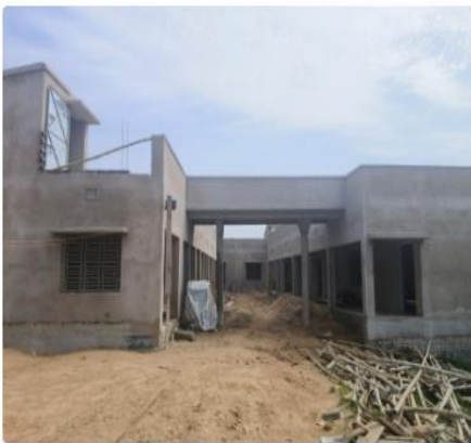
Under Construction Project
